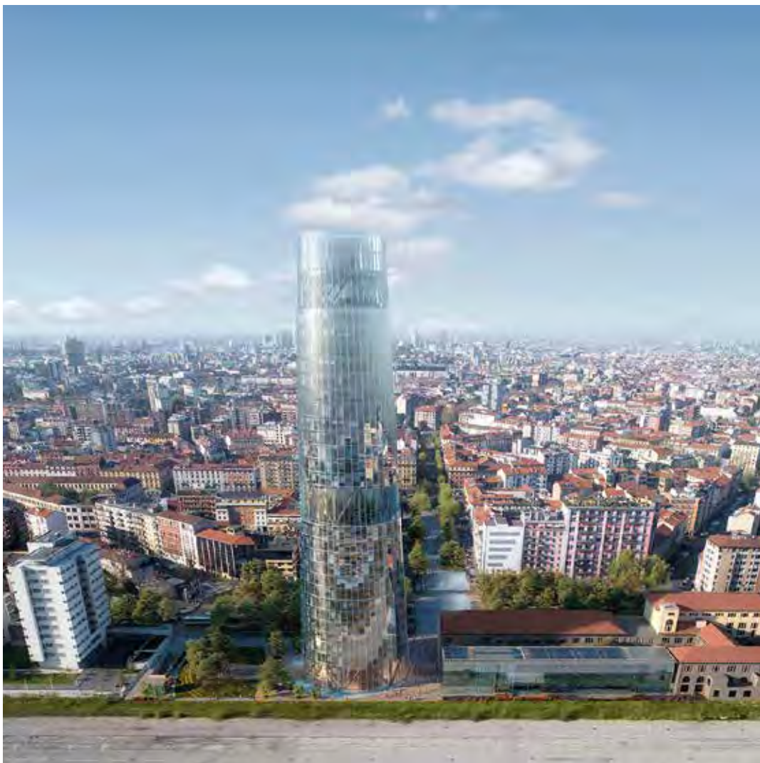
Life Tower, A2A headquarter – Milan (Italy)
