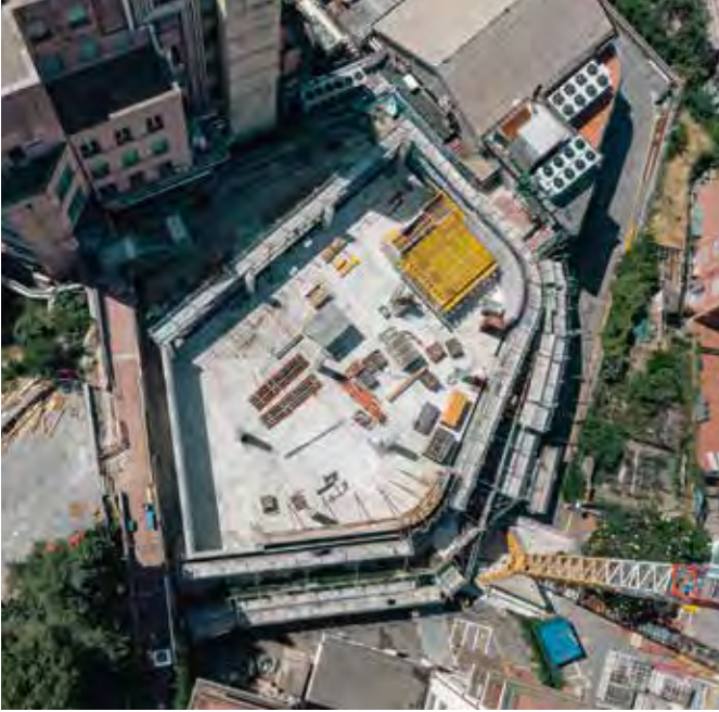
Gaslini hospital — Genoa (Italy)
