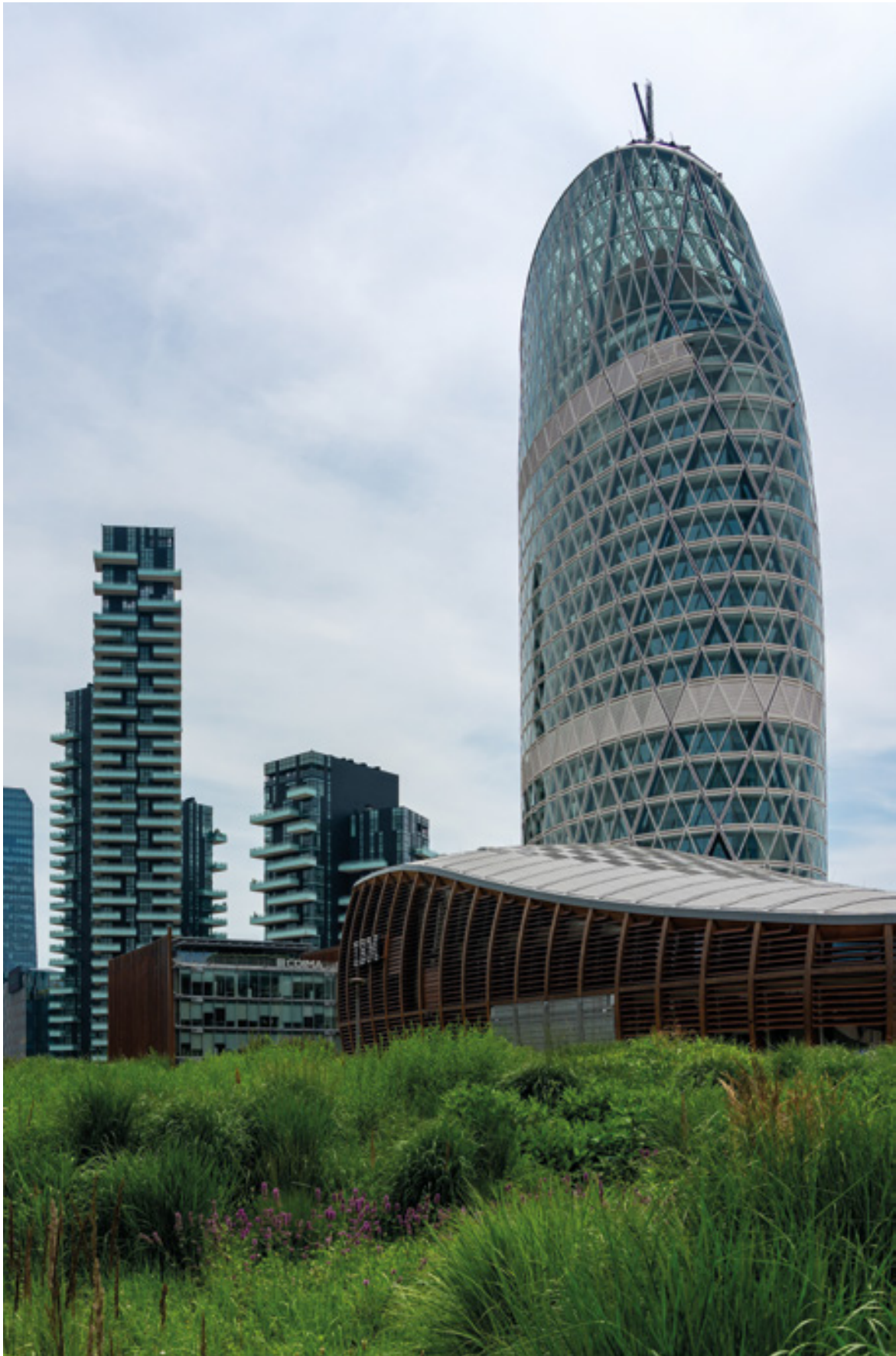
Unipol Tower — Milan (Italy)
