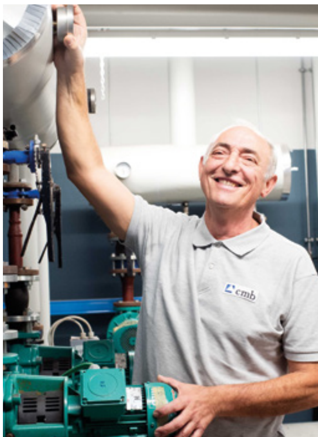
Maintenance services, Baggiovara Hospital — Modena (Italy)
