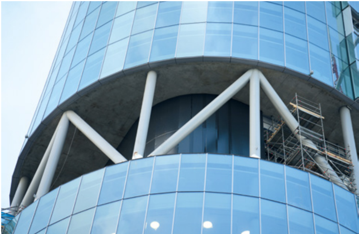
Life Tower, A2A headquarter – Milan (Italy)
