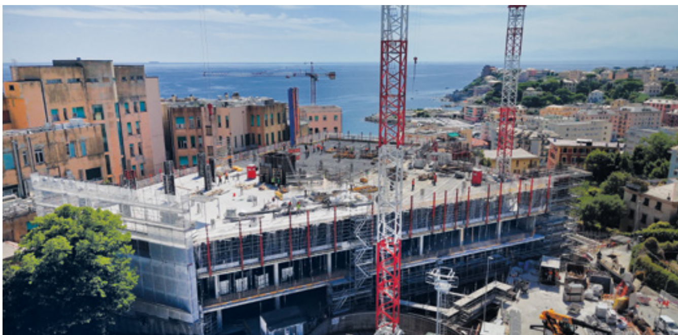
Gaslini hospital — Genoa (Italy)
