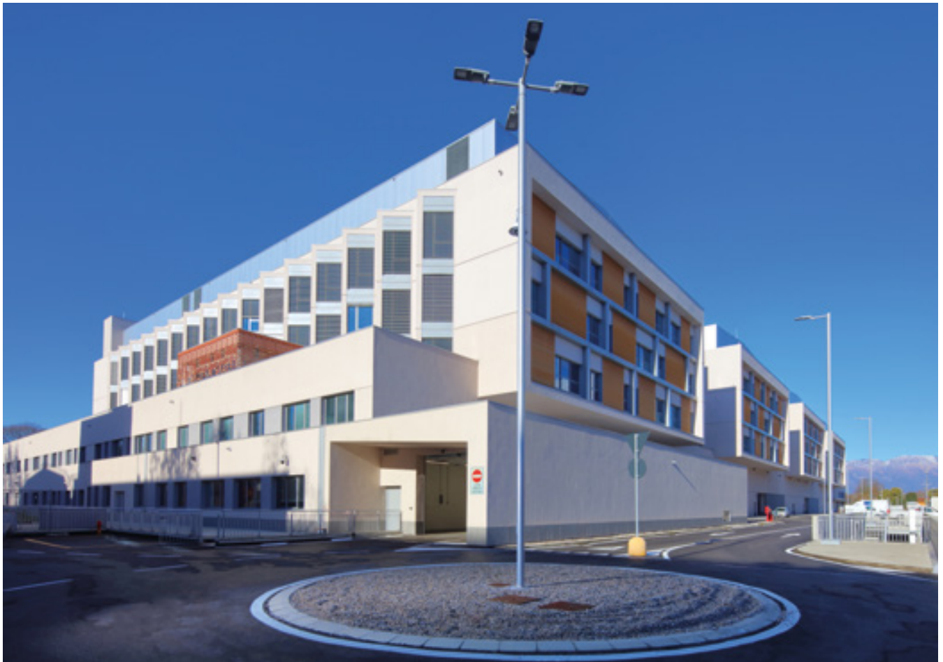
Hospital and Health City — Pordenone (Italy)
