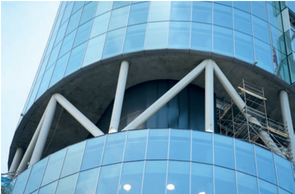
Life Tower, A2A headquarter – Milan (Italy)
