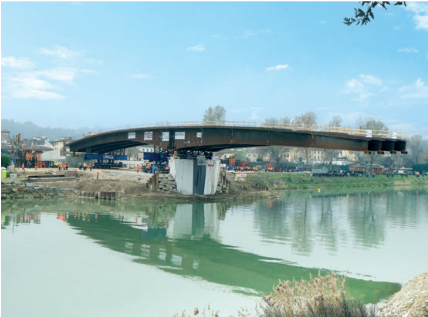
Ponte Arno Tramway lines — Florence (Italy)
