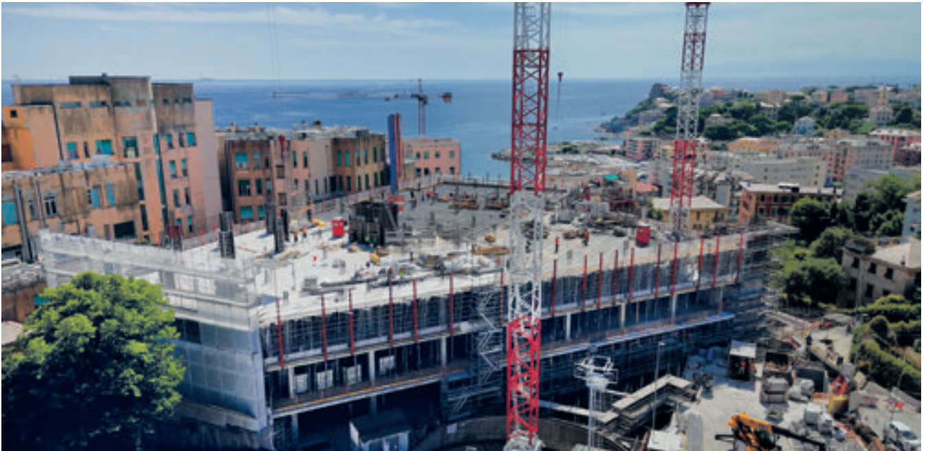
Gaslini hospital — Genoa (Italy)
